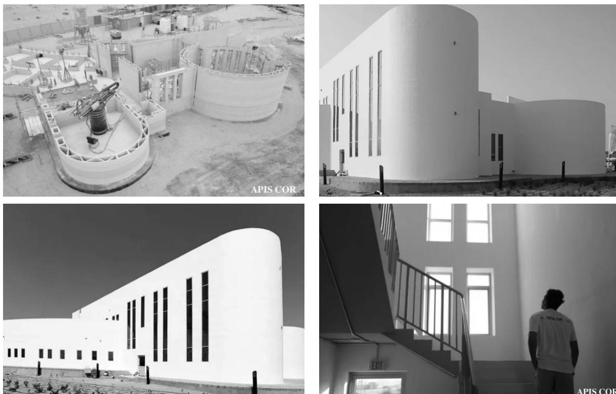
Fig. 2. The two-story building using 3D printing, Dubai
