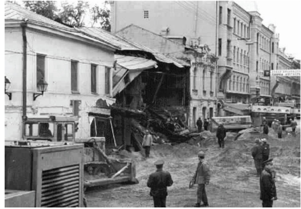
Fig. 1. A building and a street carriageway destroyed by a suffusion collapse sink formed as a result of hydraulic failure of water-saturated sands and their removal into a tunnel under construction (Moscow, 1998). Photo by V.P. Khomenko
