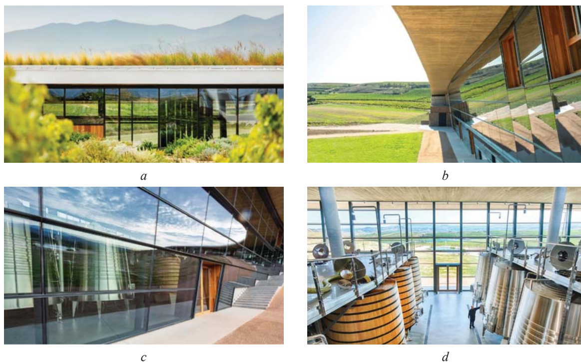
Fig. 1. Architectural solutions of Beronia winery, Spain (IDOM architects): a — part of the facade; b — facade glazing; c — exterior; d — interior 1
