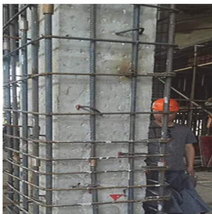
Figure 1. Concrete jacketing
