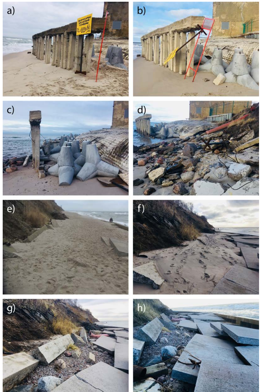
Figure 3. Dynamics of the destruction of engineering structures and the slope in the village Yantarny: (a–d) at the pumping station; (e–h) – near the bank-protective retaining wall: (a) and (e) – January 4, 2022; (b) and (f) – January 18, 2022; (c) and (g) on January 23, 2022; (d) and (h) on February 11, 2022.
